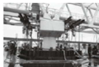
仮締切鋼板圧入状況 ▶P.15
